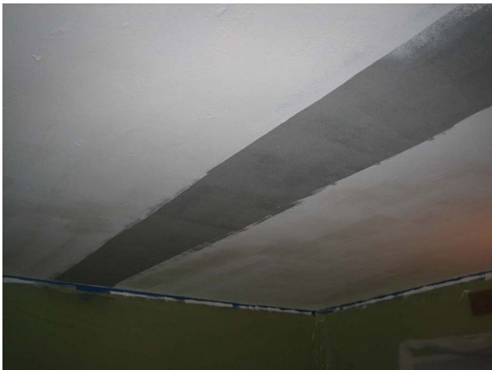
The cool blue stripe above is the area of the ceiling painted with CeraTherm GVK radiant barrier coating.
