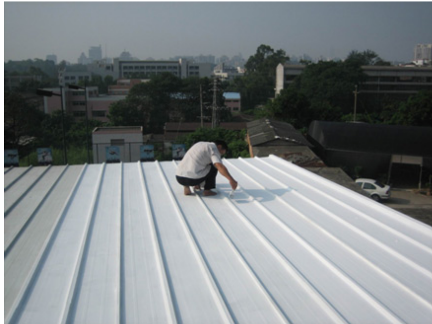
Painting the rooftop
