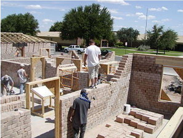
Construction method is simple. Less skilled labor is required; wall construction can be done with unskilled labor encouraging self-sufficiency and community involvement. If the blocks are stabilized with cement and/or fly ash, they can be used as bricks and assembled using standard masonry techniques of brick-laying.
